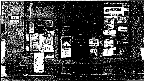
Window advertisements have eliminated almost all natural surveillance from the outside of this business, making it more vulnerable to crime.
